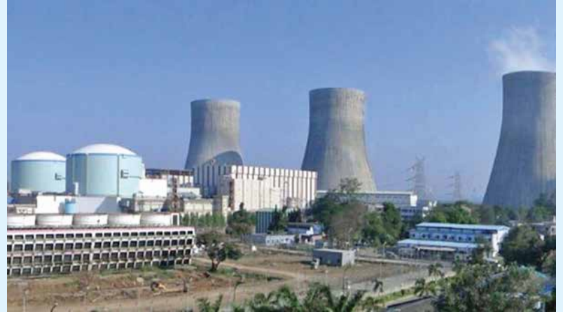
Moving forward: The third and fourth nuclear reactors with their containment domes (extreme left) at Kakrapar in Gujarat. Their cooling towers are visible. NPCIL
